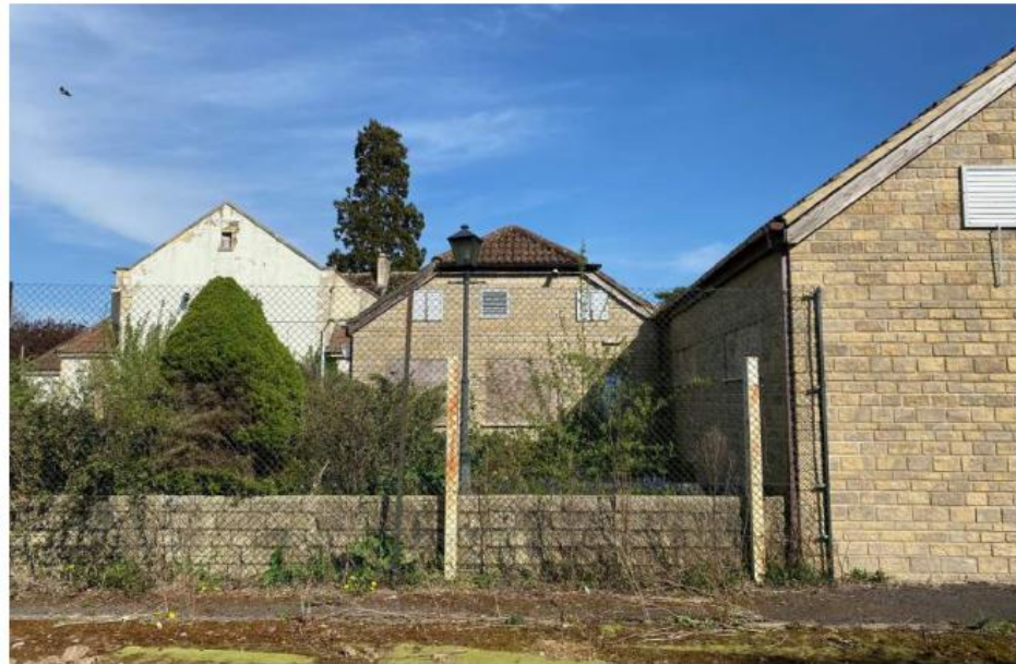
Rear elevation, 1920 hall extension (far left) and modern extensions (centre and right)
